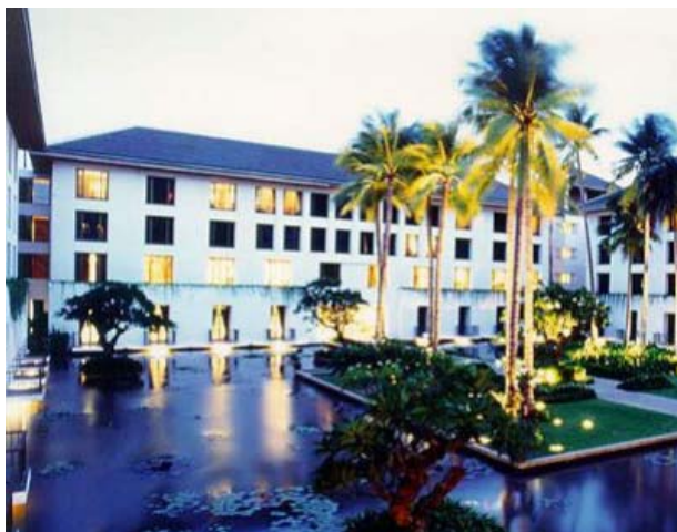
Basement, Swimming Pool & Water Tank Waterproofing
