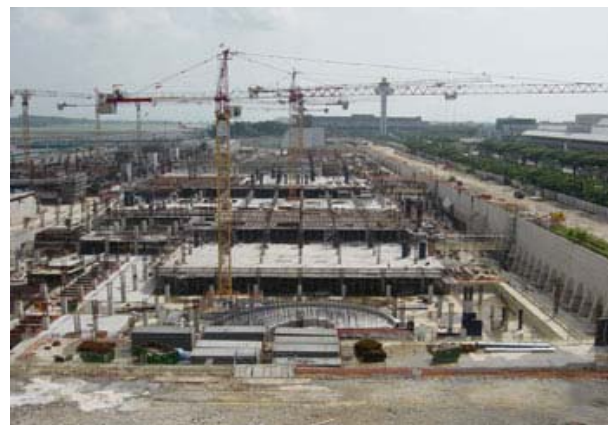
Basement Waterproofing Wastewater & Potable Water Tank Waterproofing
